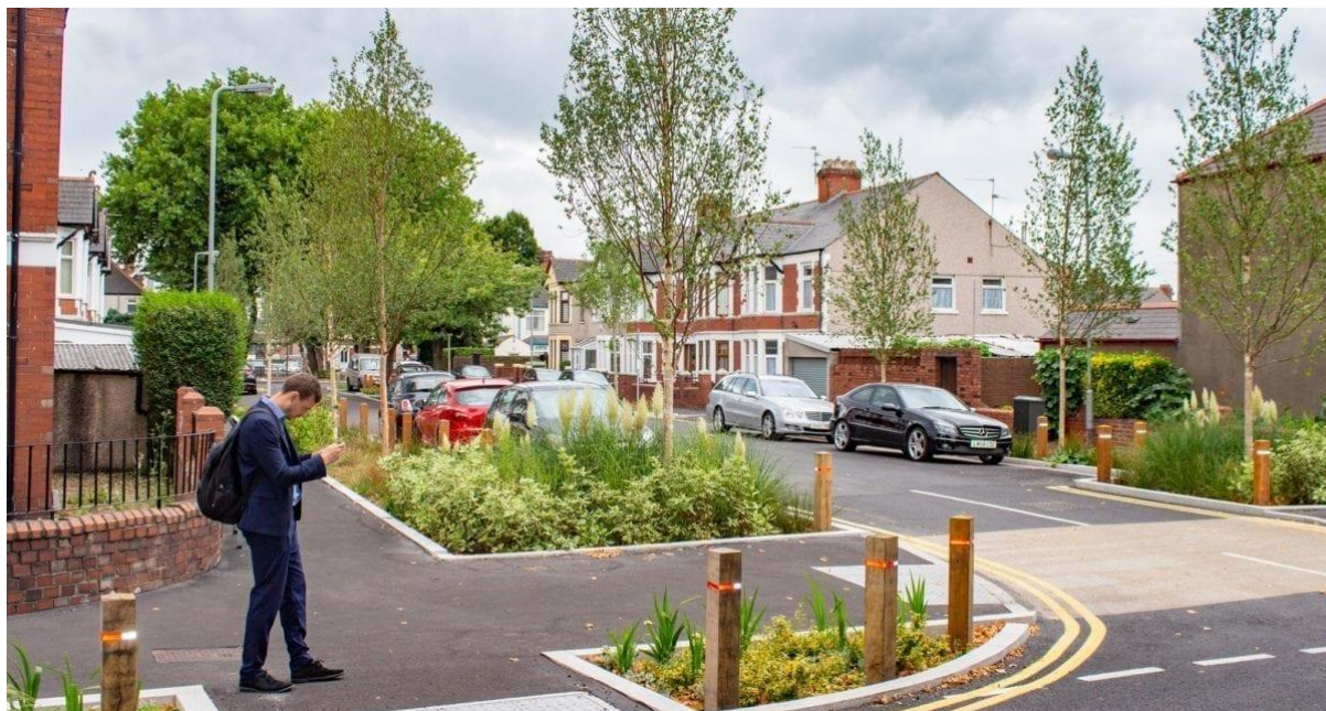
Figure 6: Greener Grangetown, Cardiff. Example of integrating green infrastructure and in an urban/residential area to promote air quality and biodiversity benefits. The scheme was led by City of Cardiff Council as the client, in partnership with Dŵr Cymru Welsh Water and Natural Resources Wales (Source: Greenblue.com and Arup)
