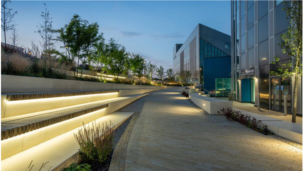
Figure 4: Sustainability focussed Newcastle Helix urban regeneration scheme - hard landscaping, amenity and accessibility detail. Newcastle Helix is a joint venture between Newcastle City Council, Newcastle University and Legal & General (source: gillespies.co.uk)
